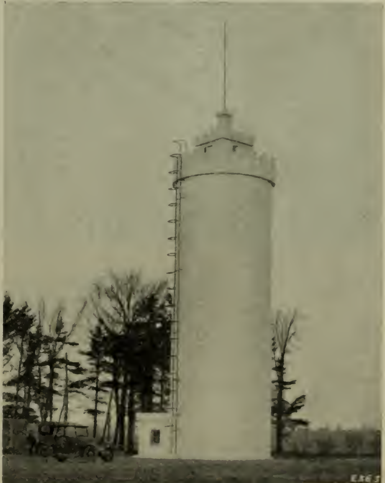
A CONCRETE WATER TOWER AT LANGSTAFF, ONT.
